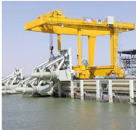
Figure 2. Hydromatrix®: in case of flood conditions, inspection or maintenance, some or all of the modules can easily be removed using a small crane.
